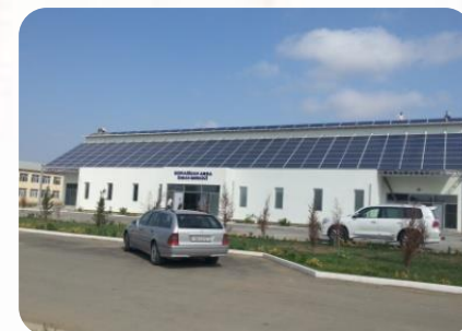
Sports Complex in Masally district (70 KW electric, 90 KW heating)
