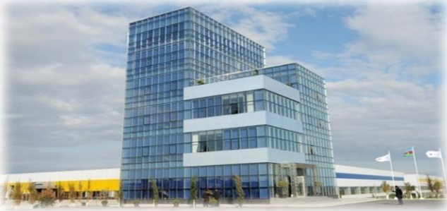
Opening of new factory - Sumgait, "Azguntech" solar panel factory
