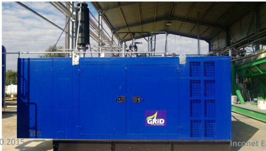
Gas Engine, Special Construction for H 2 Rich Gases
